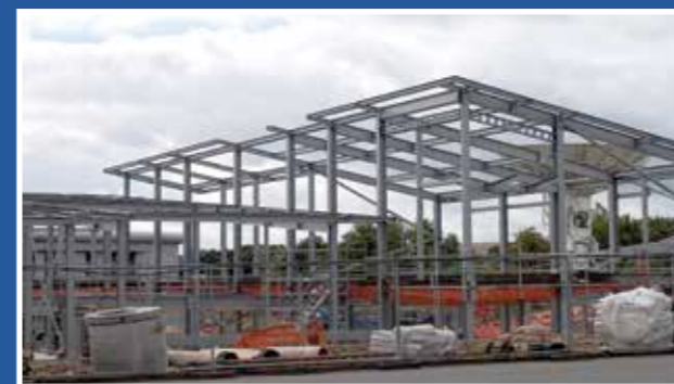
New beamline construction. Credit: STFC
