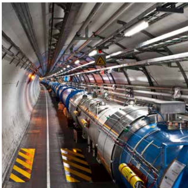
LHC Tunnel (Credit: CERN)
